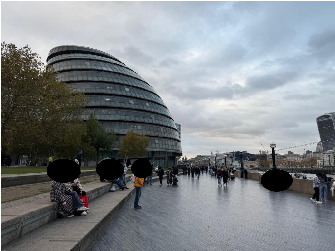
View of western elevation and the footpath in front of the site.
